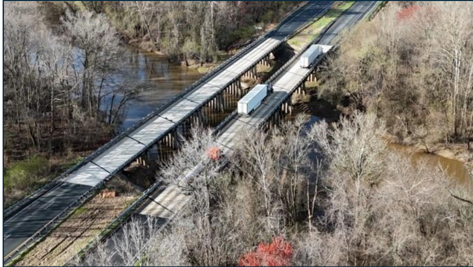
Bridge Nos. 000000001010100 and 000000001010101 over Neuse River
